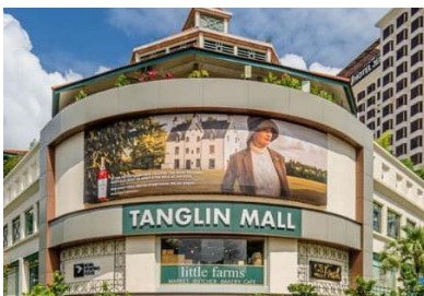
Cold Storage at Tanglin Mall
